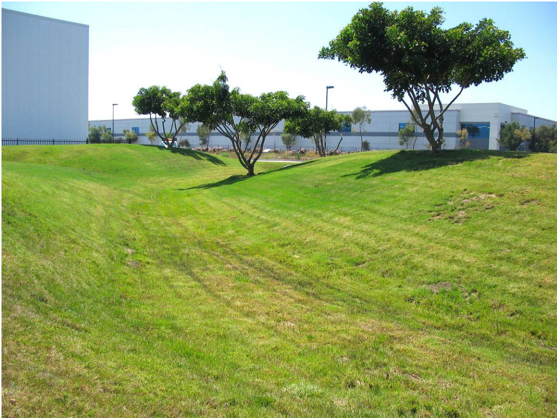
Low Impact Development Grass Swale at an Industrial Site in Oxnard
