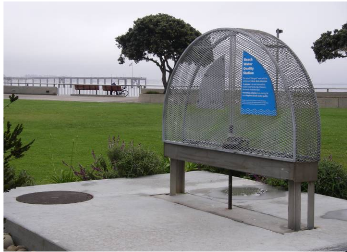
The City of Ventura's Figueroa storm drain diversion with educational signage.
